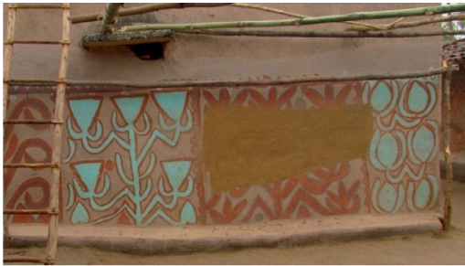
Fig.E.4: the painted wall is repaired with mud
