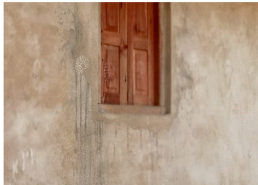
Fig E 9: white painting outside a plastered house
