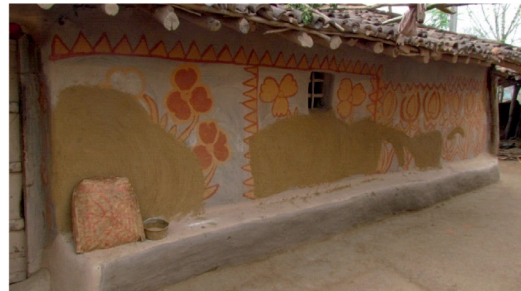
Fig.E.5: the painted wall is repaired with mud
